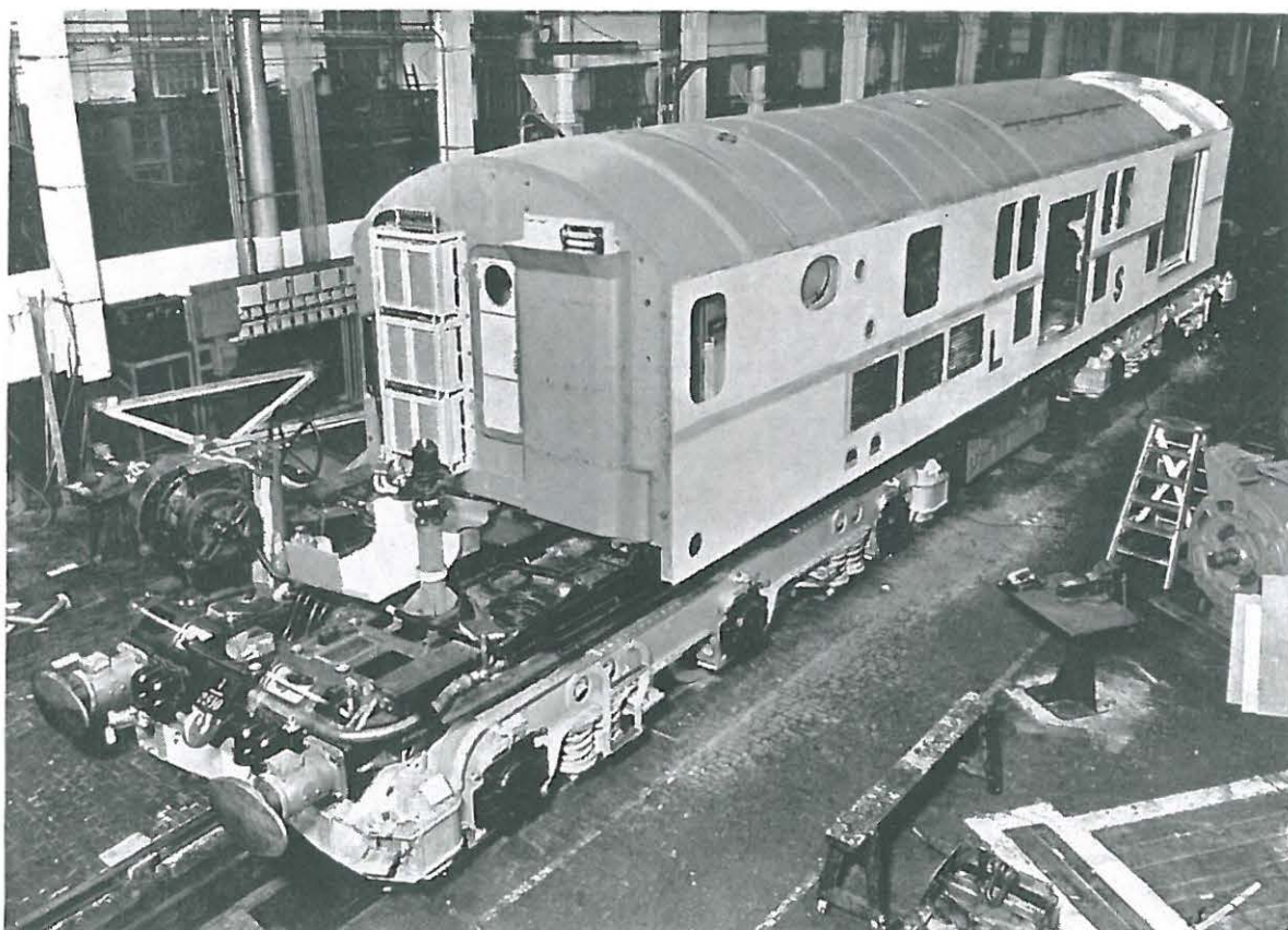
Fig. 4 Locomotive approaching completion showing motor bogies and centre superstructure in position
