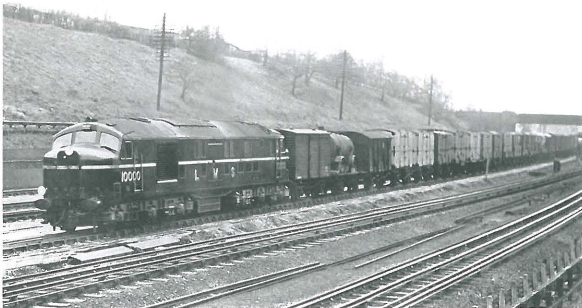
Fig. 9 In freight service. Locomotive No. 10000 hauling the 2.40 p.m. Camden-Crewe express freight train
